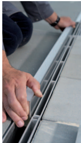
Mounting the LED elements in the slotted frame
